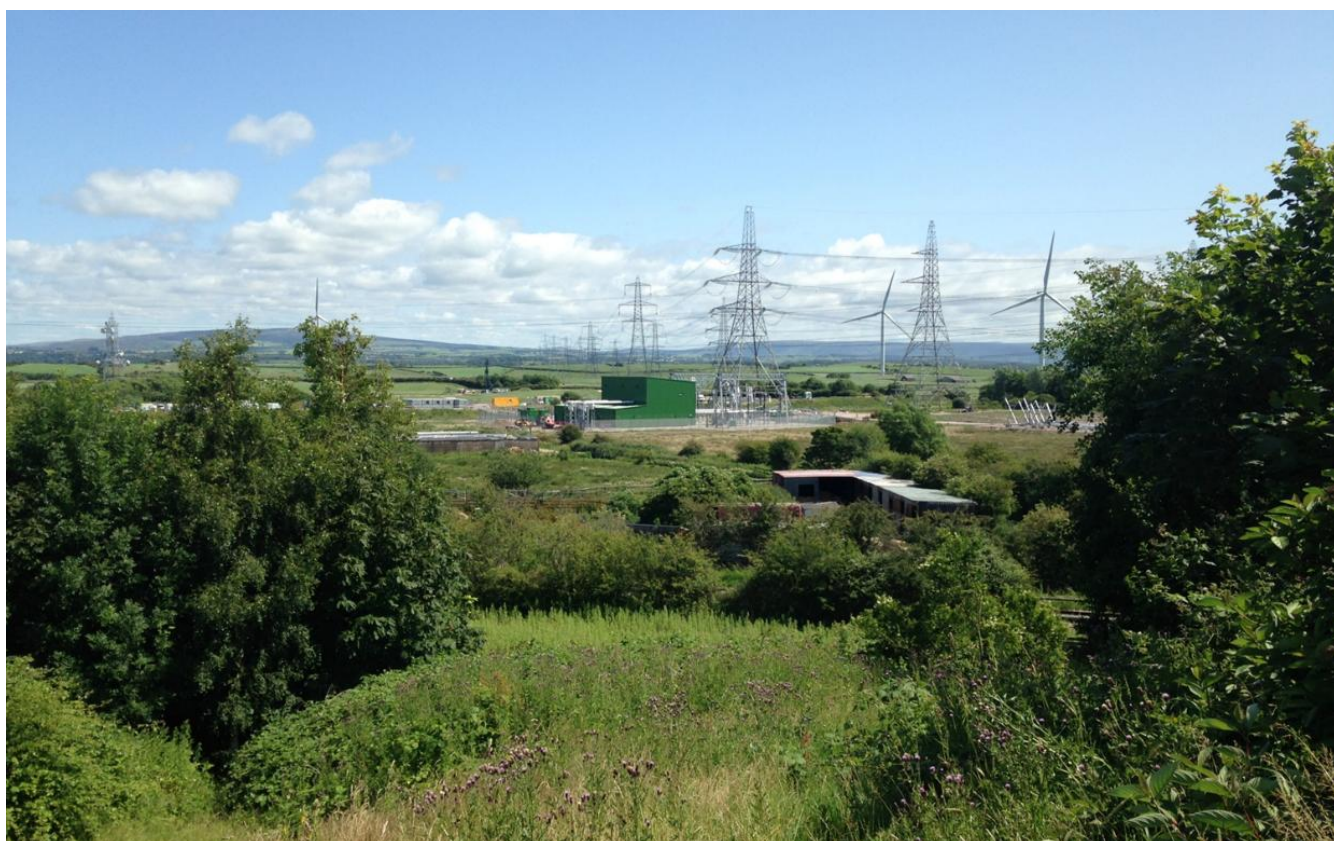
Image 3.5 Existing Middleton 400 kV Substation (Source: National Grid)
