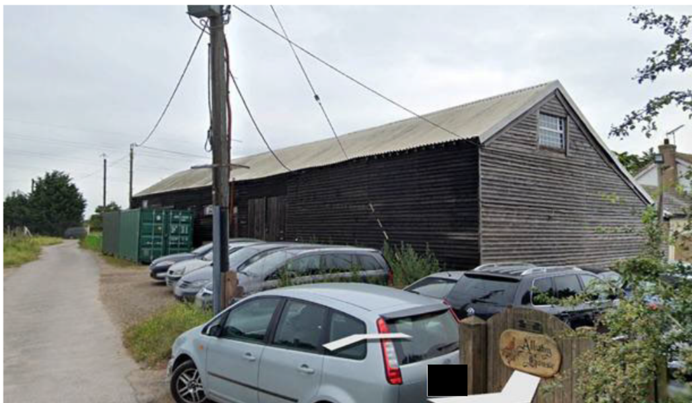
Image 5.1 Example of a building to the north of Orsett Golf Course (Source: Google Streetview 2025)
